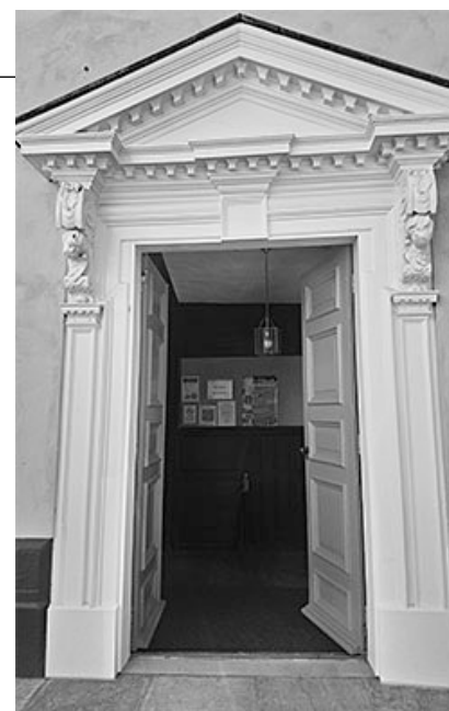
No step down into the building now.
