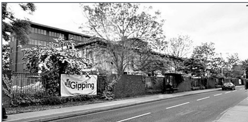
New housing coming in Handford Road.
