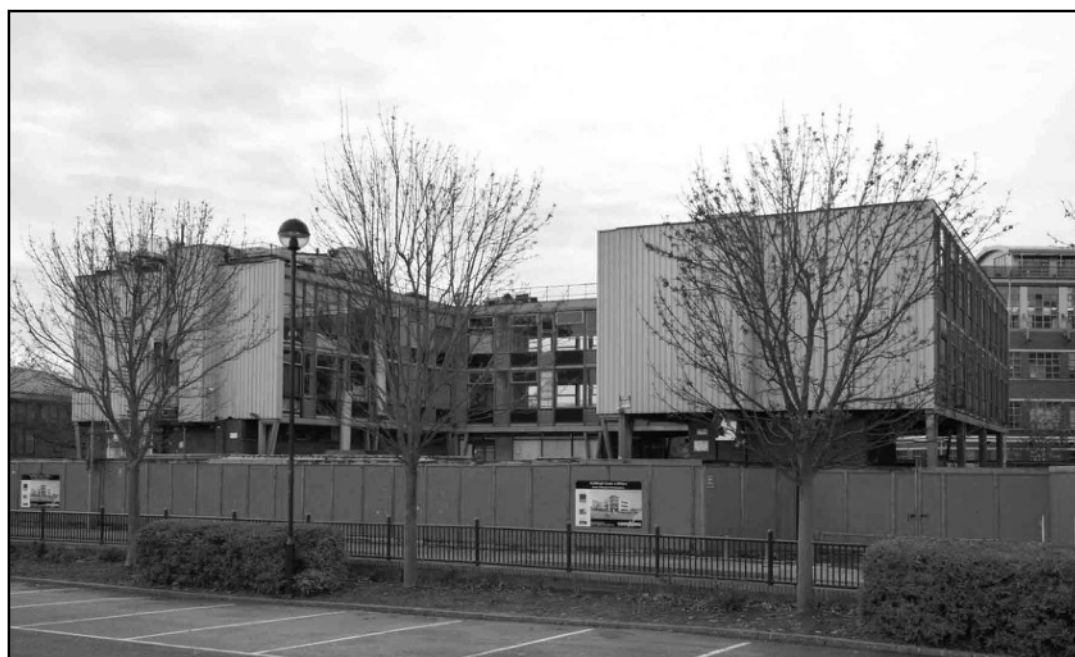
The unfinished end of the building – the fourth wing was never built – with its corrugated metal walls (photograph by John Norman, 2015)
