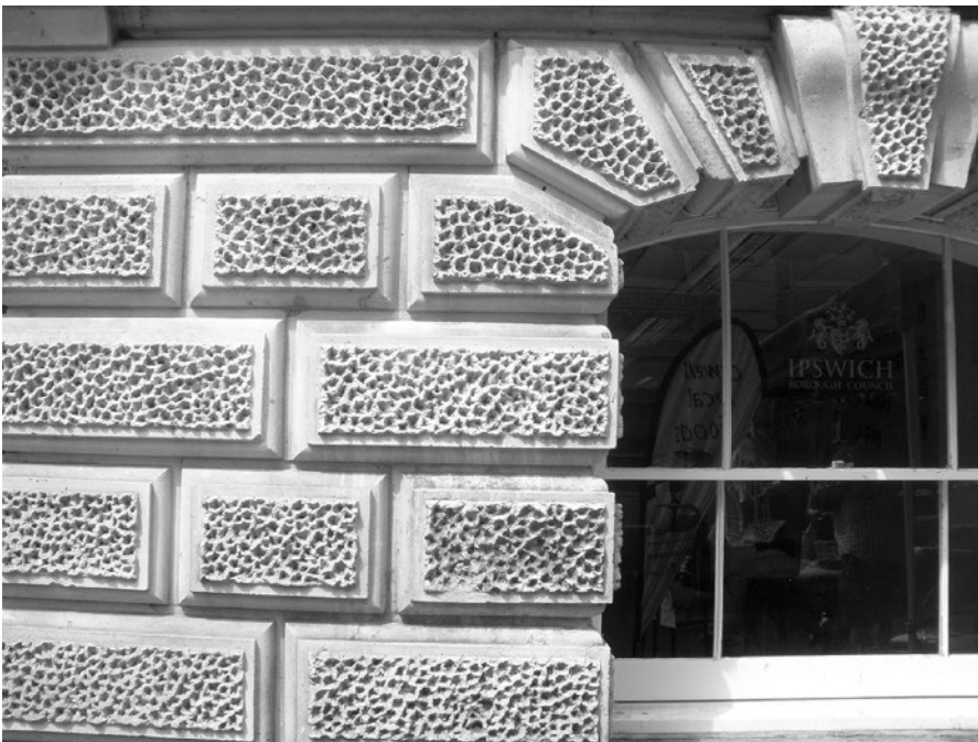
Masons have enhanced this Bath Stone on the Town Hall with a honeycombed surface, copying the weathered burrowed surfaces occasionally seen in other limestones.
