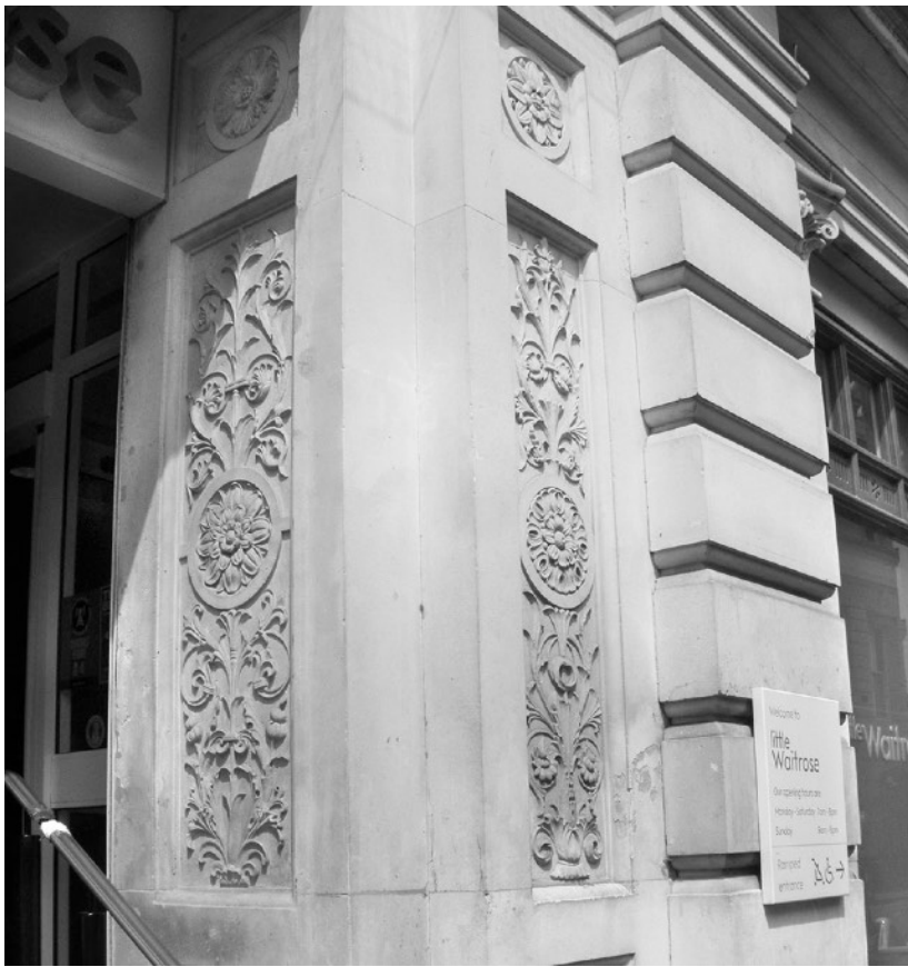
Fine-grained Portland Stone can be carved in any direction and hold fine detailed work as here at the entrance to Waitrose in the Corn Exchange. (Photographs by Bob & Caroline Markham)
