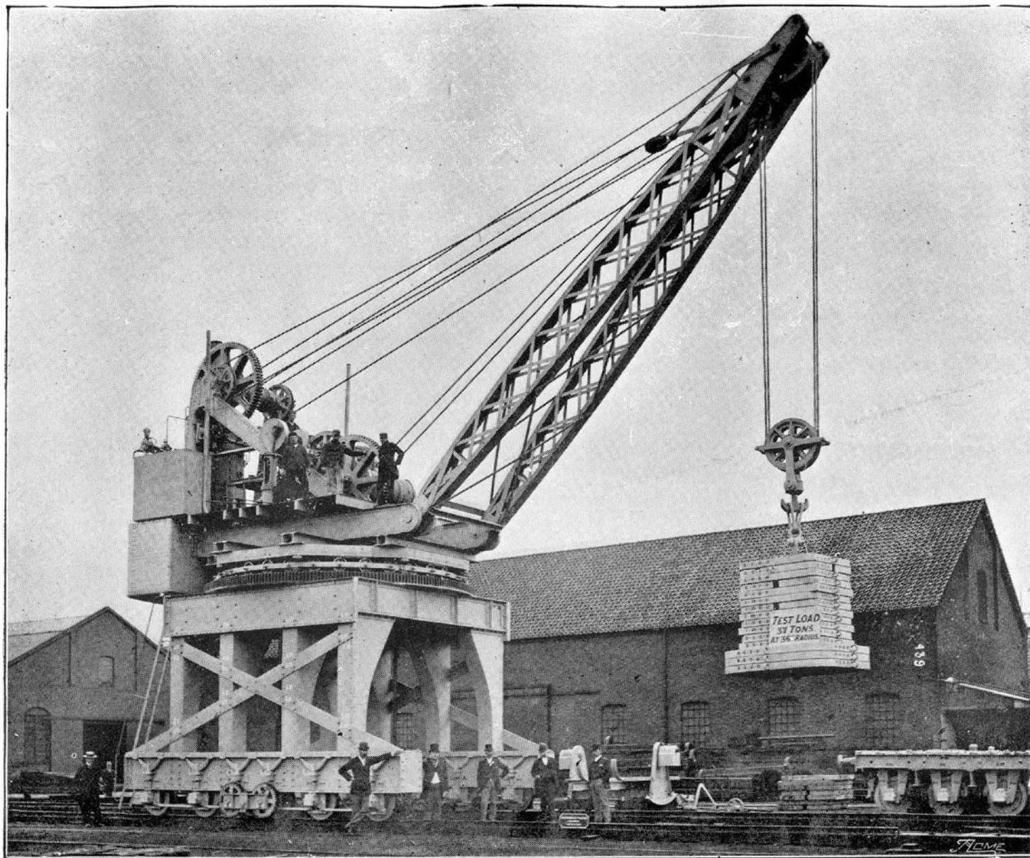
37 ton Crane built by Ransomes & Rapier, Ipswich, for the Great Eastern Railway Co. Special Flexible Steel Wire Ropes supplied by THOS. & WM. SMITH.
