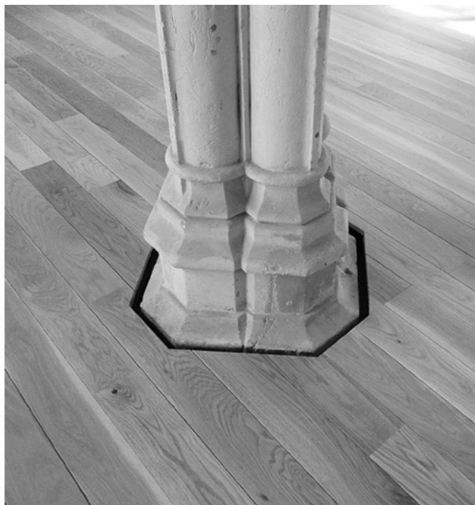
Details of the St Clement renovations showing repaired plasterwork on the interior of the south wall and the cluster of pillars emerging through the suspended floor. The project cost around £150,000 including fees plus VAT. The contractor was F.A. Valiant & Son, specialists in the restoration and conservation of churches.
