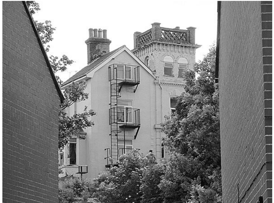
The Warren (Rotherham House) taken from below in Samuel Court. The top of the fire escape was my sitting room and the top windows of the tower were my bedroom, with access to the roof through a hatch. The view is fantastic and could command 'penthouse suite' status if properly refurbished.
