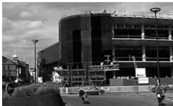
The Willis Building under construction 1974-5
