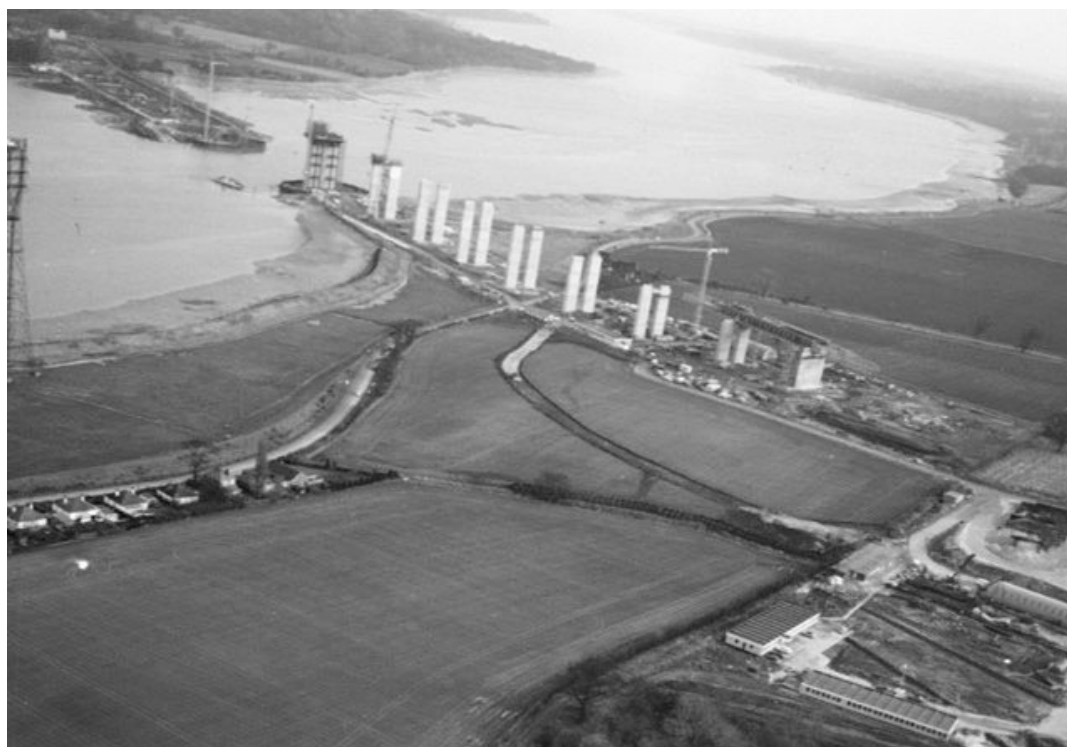
The Orwell Bridge starts to take shape; photo by Brian Mateer.
