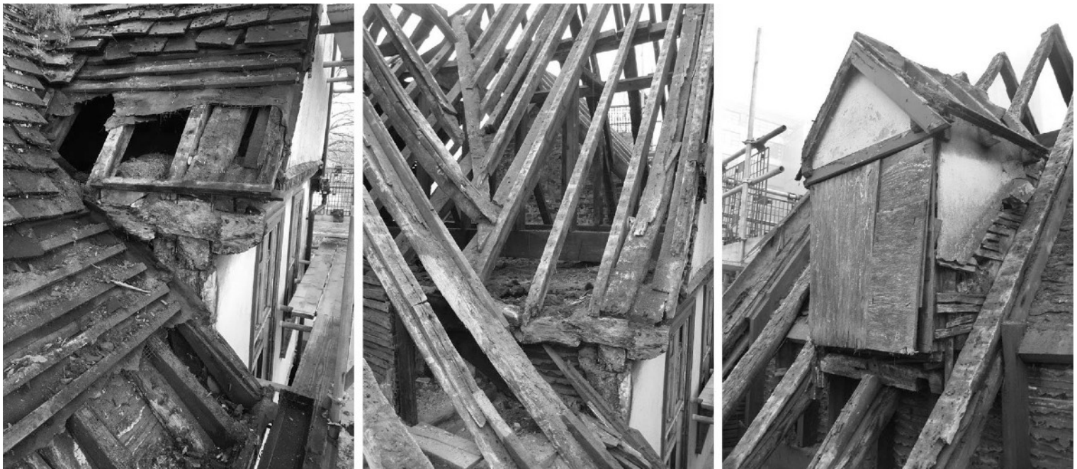
Roofing works on gable and dormer window.
