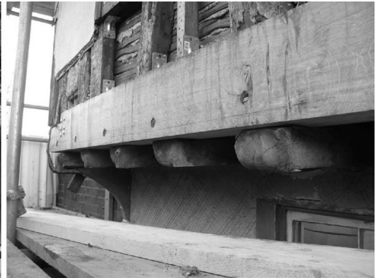
Strengthening and renovation.
